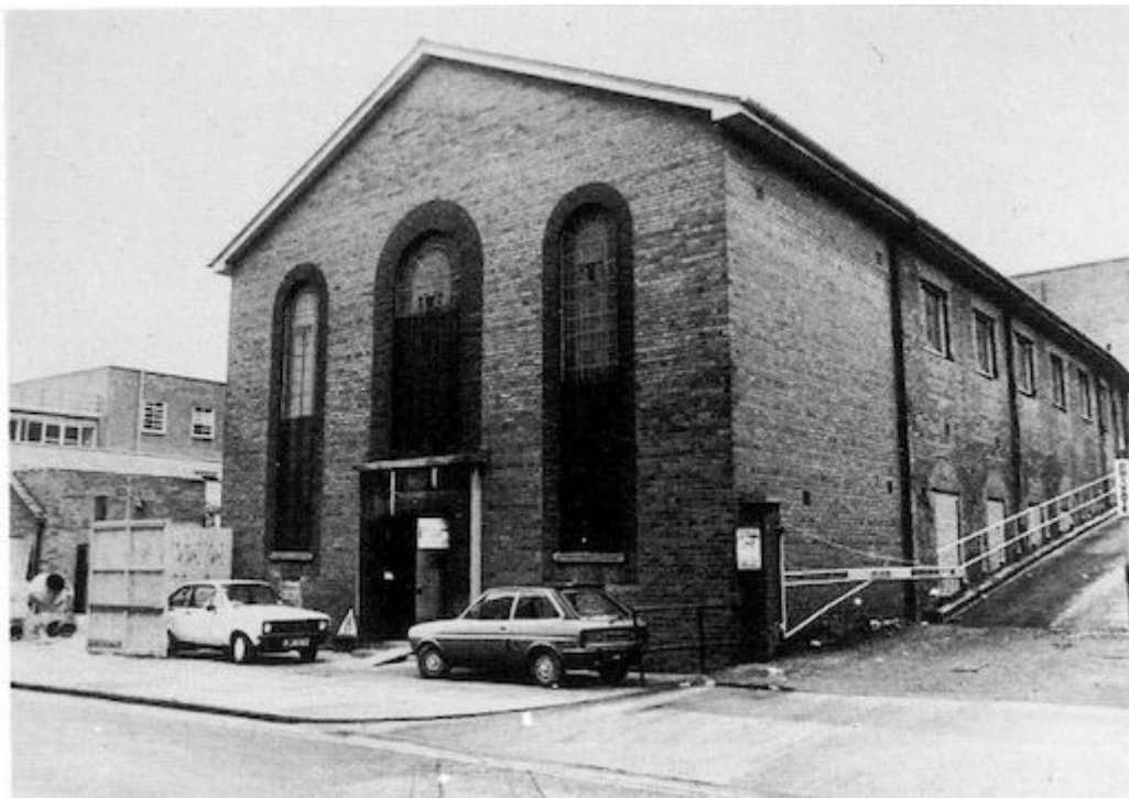
Hull Old Hebrew Congregation Osborne Street, from 'Lost Churches and Chapels of Hull' by David Neave, 1991
